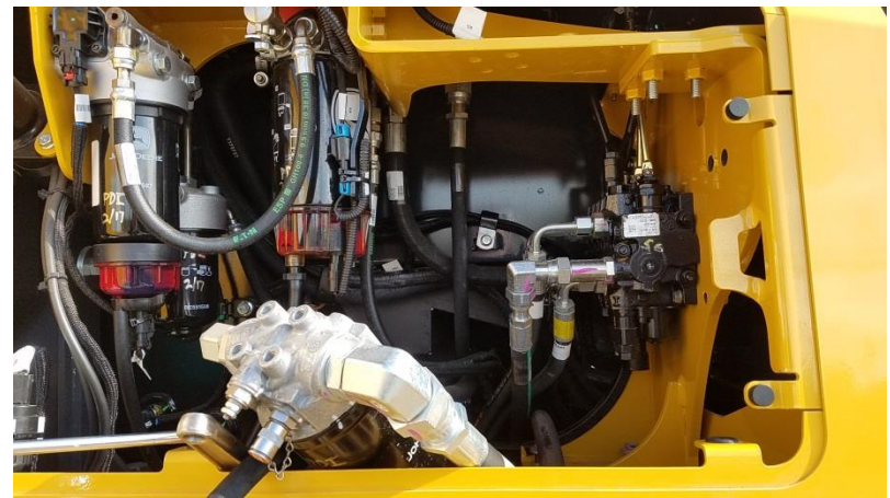
Fig. 5 - Hydraulic Oil Filter Removal
