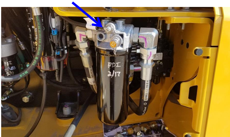
Fig. 4 - Hydraulic Oil Filter Removal
